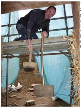
Working with straw bales has several advantages. Straw is sustainable as it's an annually renewable product, it's highly insulating (both for warmth and acoustically) and once plastered the walls are less of a fire risk than traditional timber frame. It is low cost, structurally sound and provides a healthier living environment with no associated toxins and pollutants used in conventional building construction.
